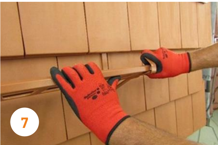
Place the grid to the rail! The overhang of the grid has to be lower than the 1/3 part of the support distance!
