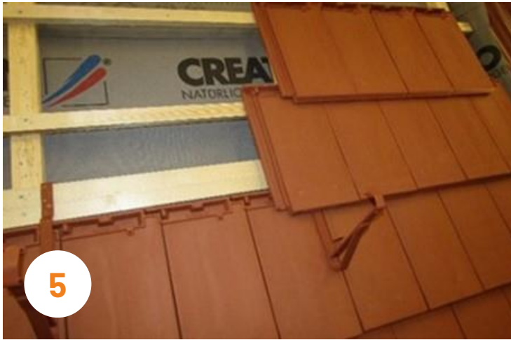
Finish the tile cover and use the ventilation tiles above the snow guard grid supports!
