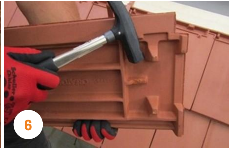
For some tile model you have to broke out one or more support in the ventilation tiles! You can find further information about this in the end of this guide!
