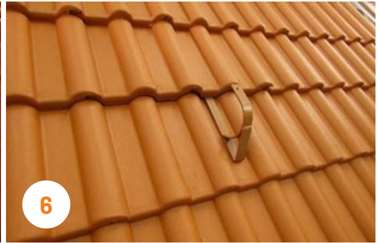
Place a base tile above the safety hook!
